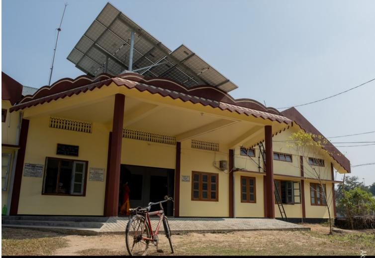
The health center now has reliable power supply through a three-phase 5 kWp solar PV system with 18 kWh battery storage. The system was installed with support from WRI India, in collaboration with HSBC India and the Catholic Health Association of India (CHAI).
