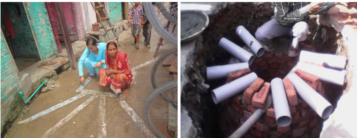
FIGURE 5 | Images from CURE's project at Safeda Basti: Simplified sewer networks to home toilets, managed by local committees
